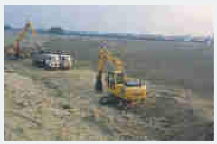
**Picture 9:** Waste Water Treatment Plant stabilizing pond earthwork excavation works in progress under Drainage Sewerage Waste
